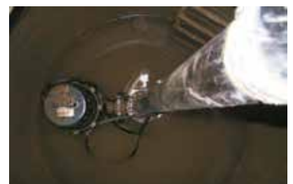
RH80 pump lowered into its installed position with delivery pipework connected
